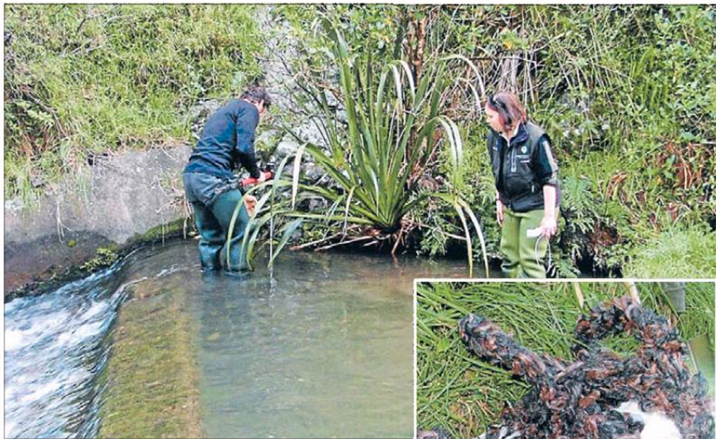
Fish ladder: Department of Conservation workers sink a stake in the Korokoro Stream bed for a rope (inset) that will help native fish 'climb' past dams and weirs.
